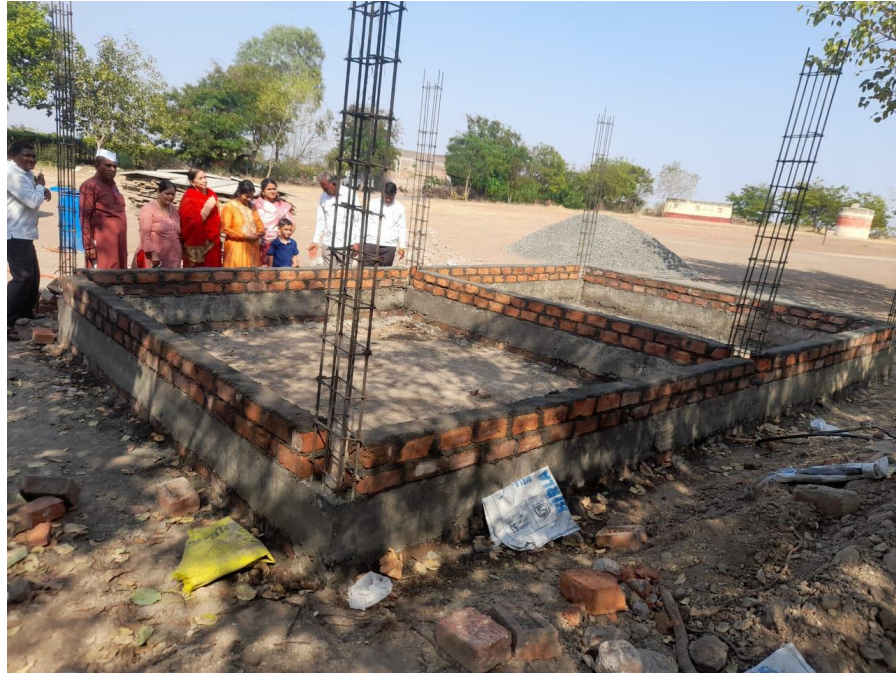
Sanitation block for students under construction at the Rameshwar Vidyalay
