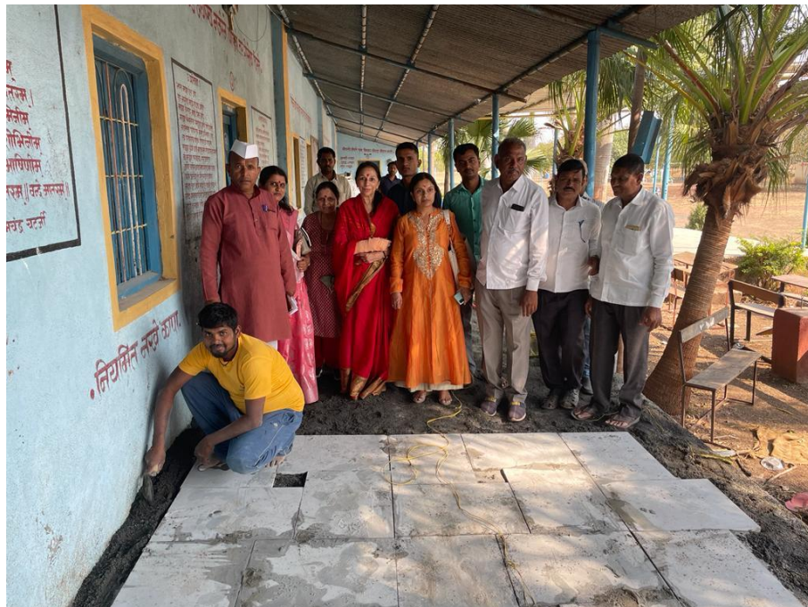
Installing stone flooring in the school corridor at Rameshwar Vidyalay
