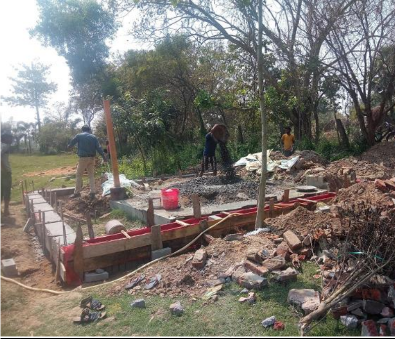
The plinth under construction at the Vidya Niketan study centre
